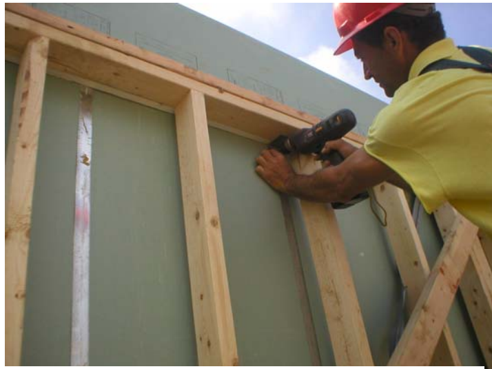
Worker attaching aluminum L-clip to steel framing on area separation wall.
